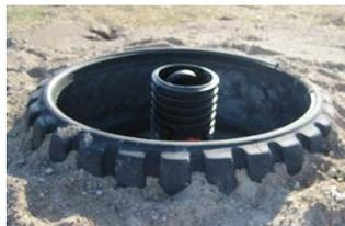
**One of the large tire water tanks installed by Brian Johnson.**
