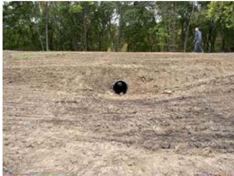
**A side water inlet offers a man-made field drain.**
